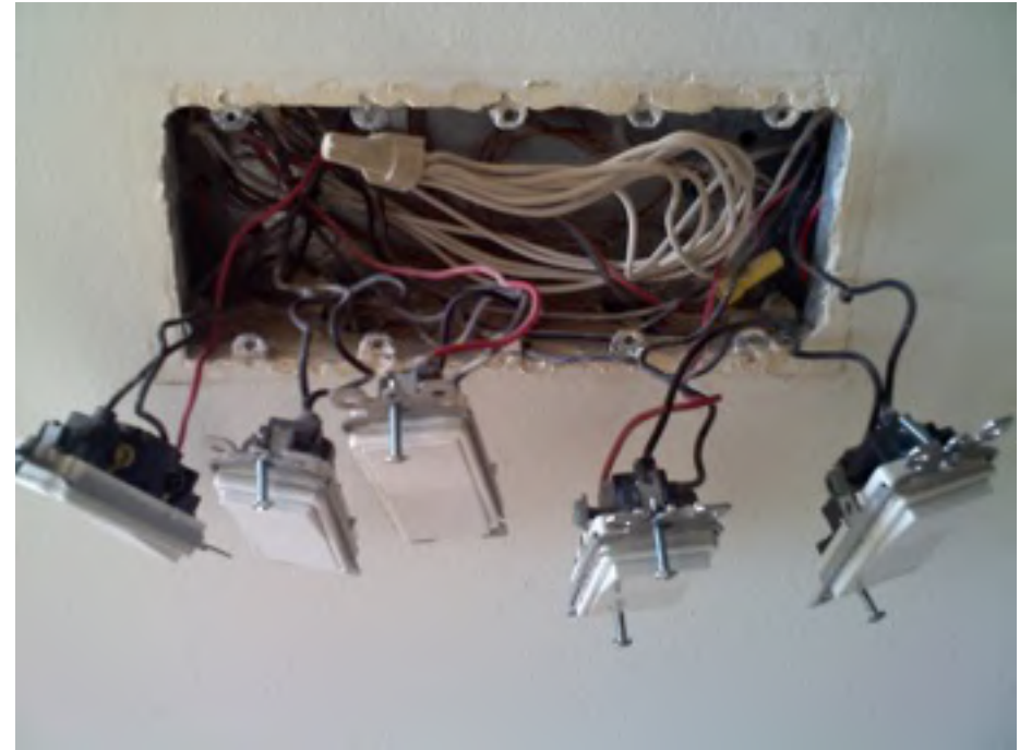
Two circuits in one junction box — Neutrals are all grouped together
