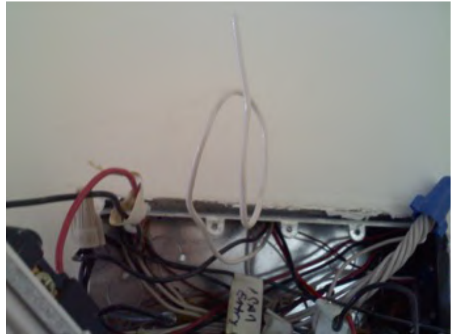
Neutral conductor not connected to any other conductor in junction box
