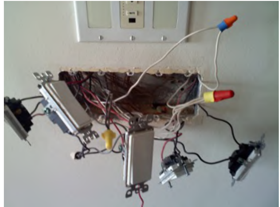
Two circuits in one junction box — Neutrals of each circuit are now separated
