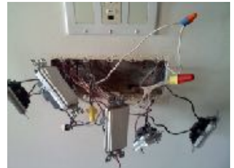
Neutrals of same two circuits, separated
