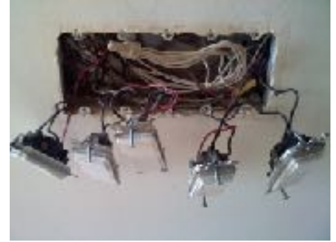
Neutrals of two circuits, combined
