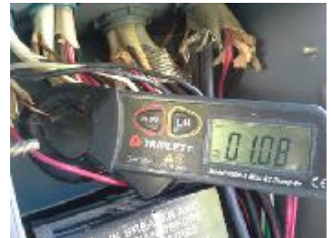
1 Amp on circuit ground, measured at panel
