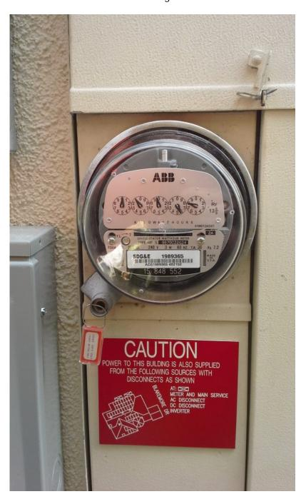
This is actually a bit unusual in that we are told by certain other electric utilities that they cannot use an analog meter, which is what smart meter opt out customers get, on a house with a grid-tied net metering system with PV panels. Yet San Diego Gas & Electric has just such a set up at this house in Ladera Ranch.
